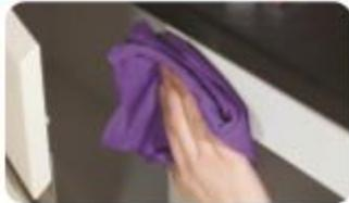
Fred adhesives are instantly strong. They cannot be repositioned when placed incorrectly so test each step first, **without** exposing the adhesive. Before installation, clean and dry the surface with a 50:50 solution of water plus white vinegar or surgical spirit.
